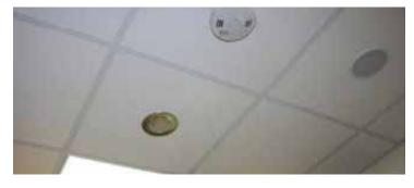
Drop ceilings help provide a professional office setting that patients expect and appreciate. They also provide easy access for the installation of new wiring and equipment. Individual panels can be cleaned and replaced easily as needed.
