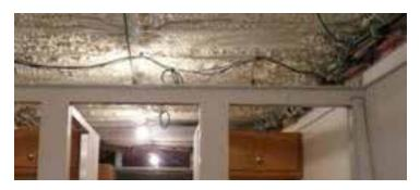
Insulation rated R12 or higher is essential to keep staff and patients comfortable while protecting sensitive equipment, such as mammography and other x-ray units. Better insulation also means less strain on your HVAC unit.
